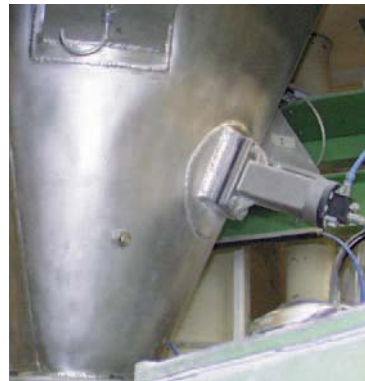
Cleaning bunker walls
