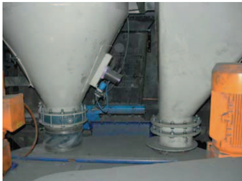
Loosening hard crusts with pneumatic linear vibrators
